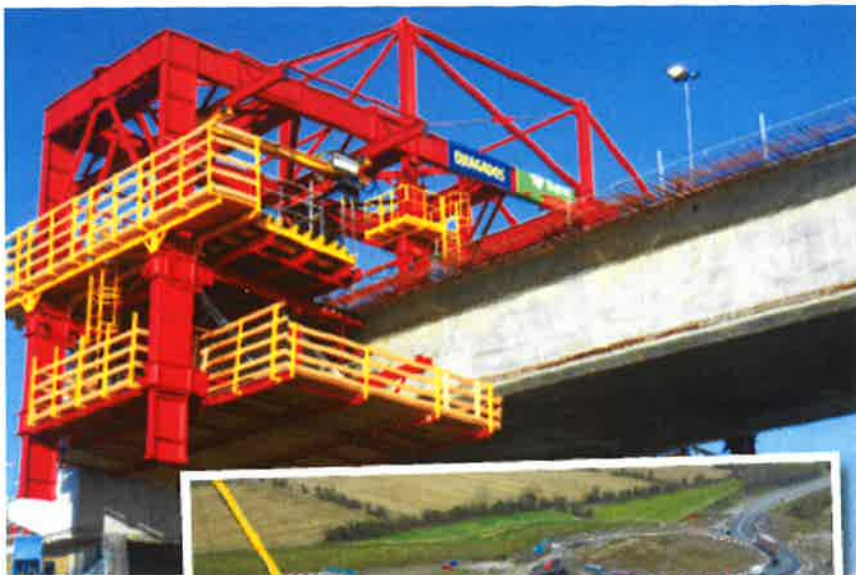
Wing Traveller – Design drawing & photo of it assembled
